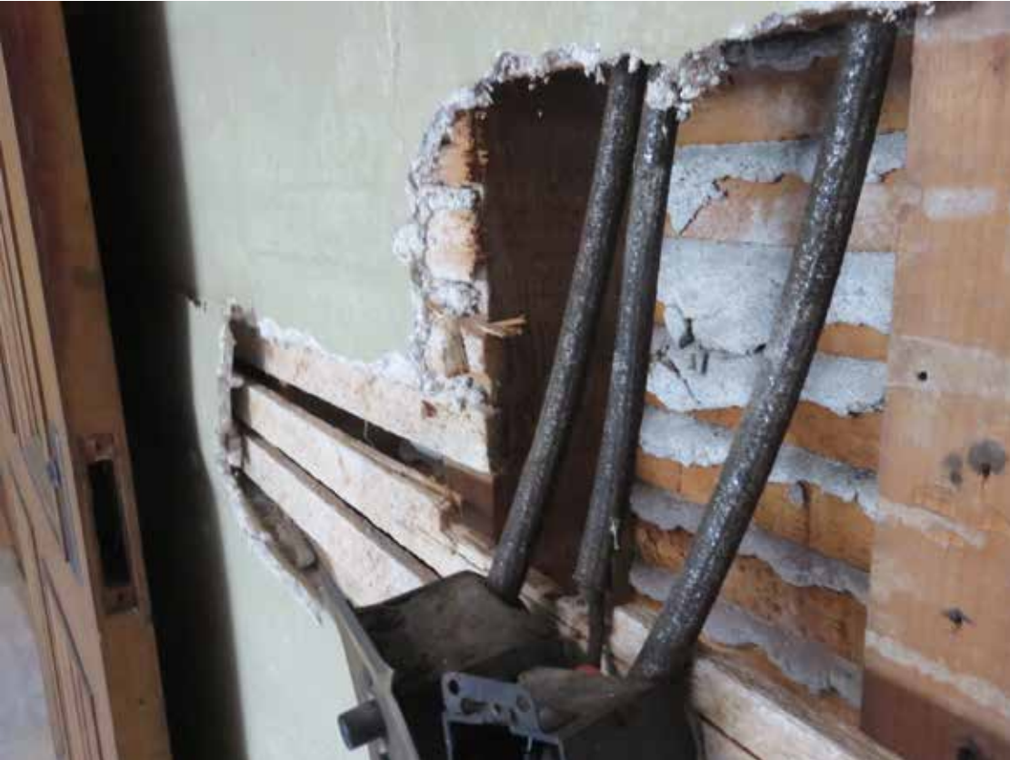
Existing wood studs with lath and plaster with original wiring
