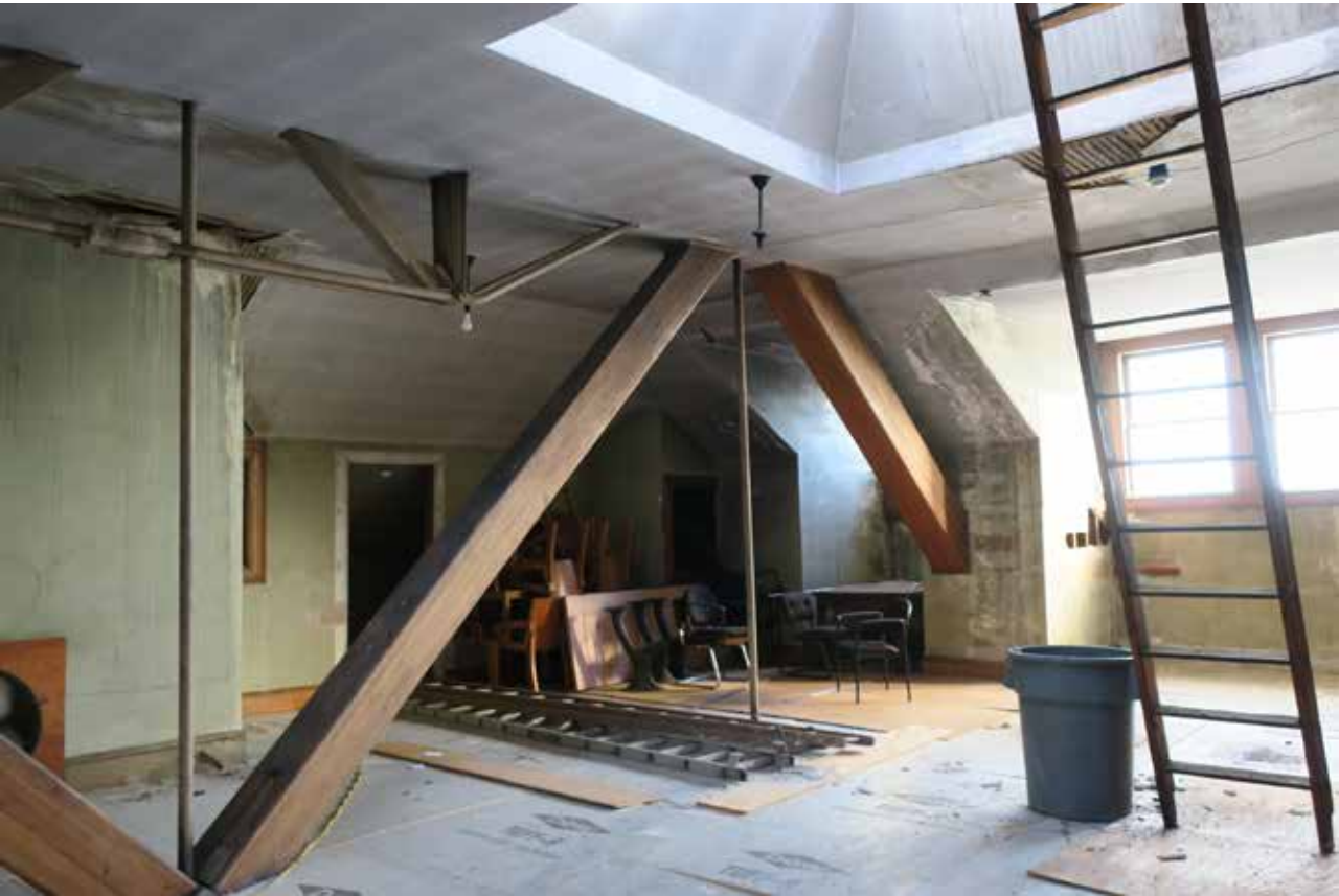
Existing heavy timber and metal trusses
