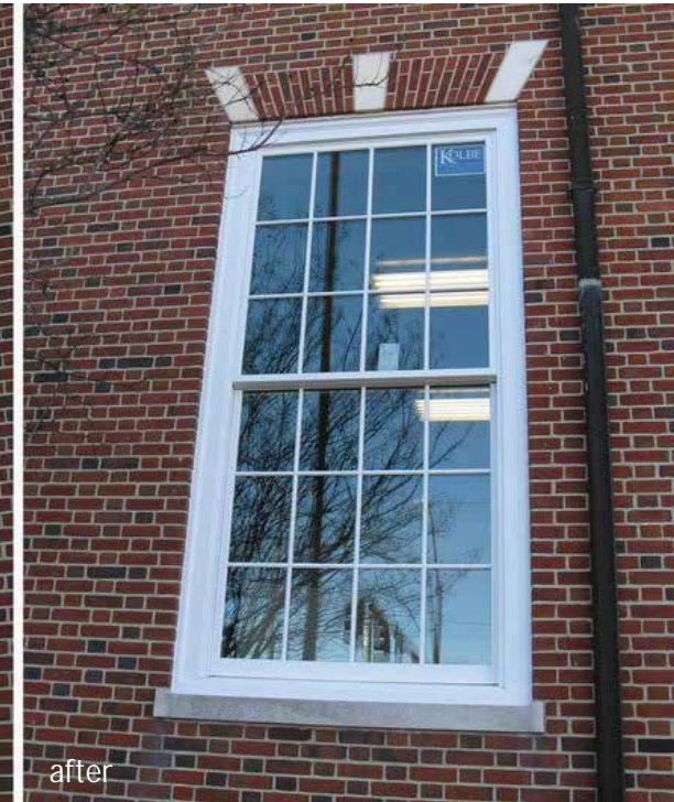
Example of Aluminum clad with insulating glass
